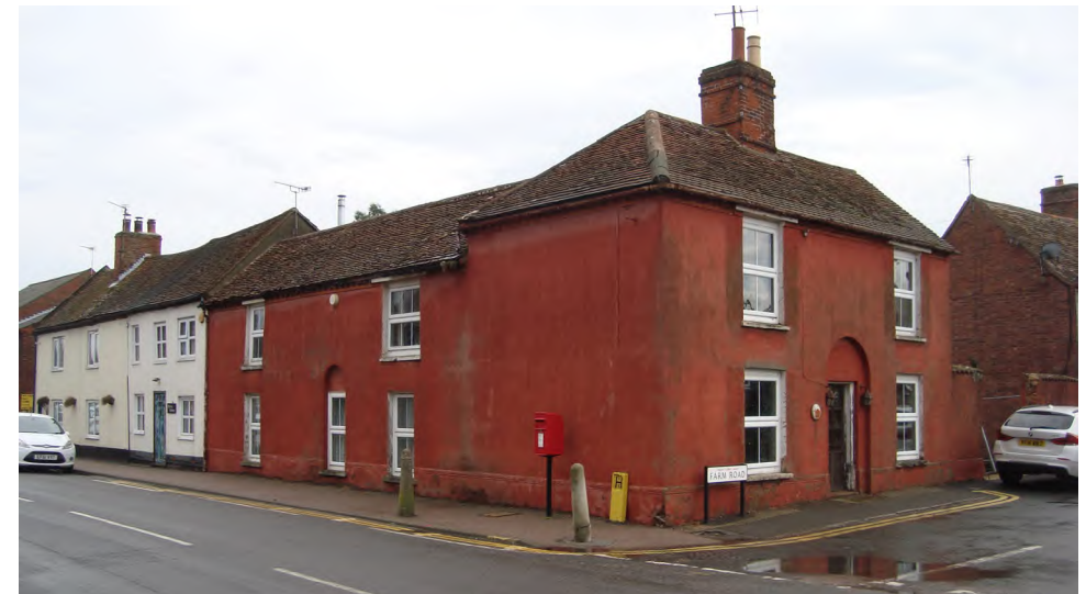
Figure 45 The insertion of inappropriate uPVC windows has harmed the historic and architectural interest of the Conservation Area
