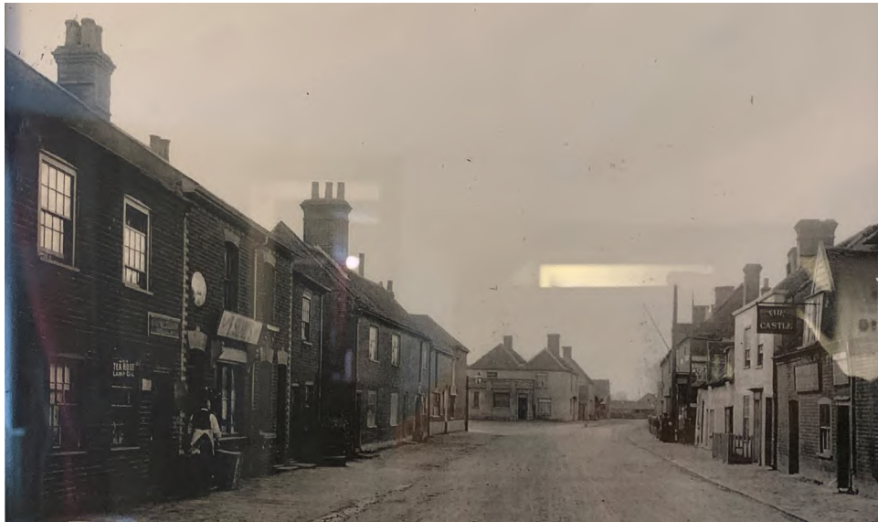
Figure 7 Historic image of Great Oakley High Street looking west c.1900
