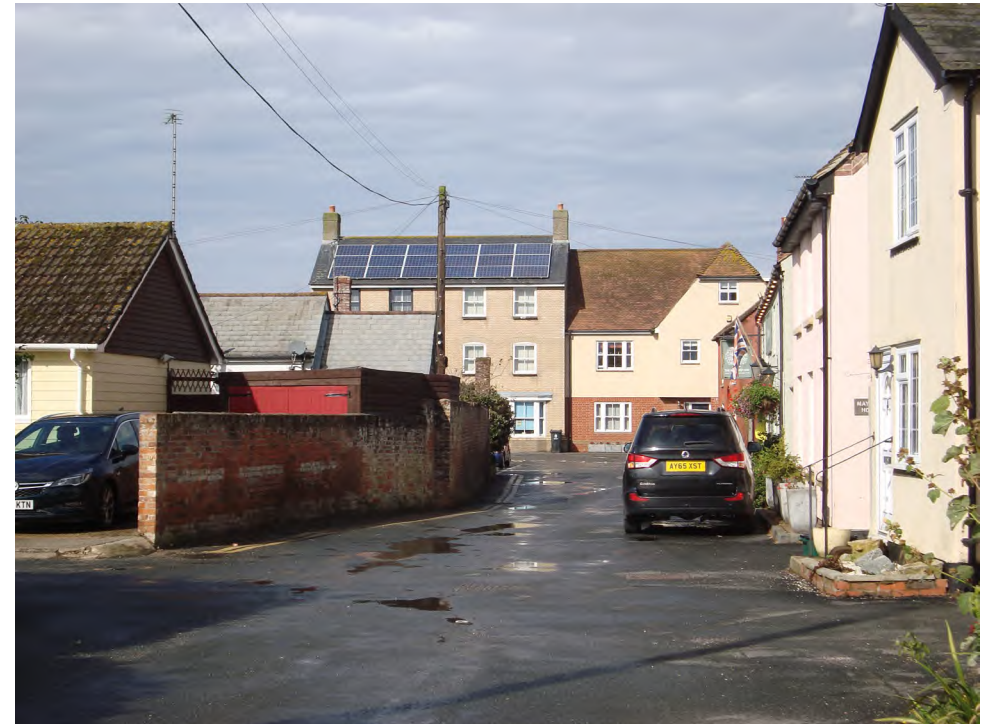
Figure 50 Solar panels on modern dwellings can be intrusive to the traditional, vernacular roofscape of the Conservation Area when applied to front-facing roof pitches
