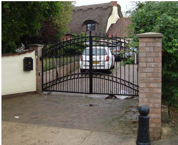
Figure 47 Inappropriate modern metal gates to a vernacular dwelling on Farm Road
