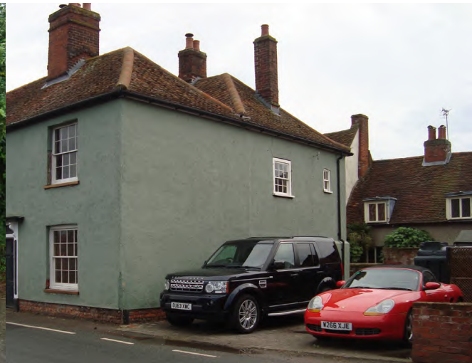
Figure 48 Removing historic boundary treatments to create parking, such as by Cambria House on the High Street, erodes the special character of the Conservation Area
