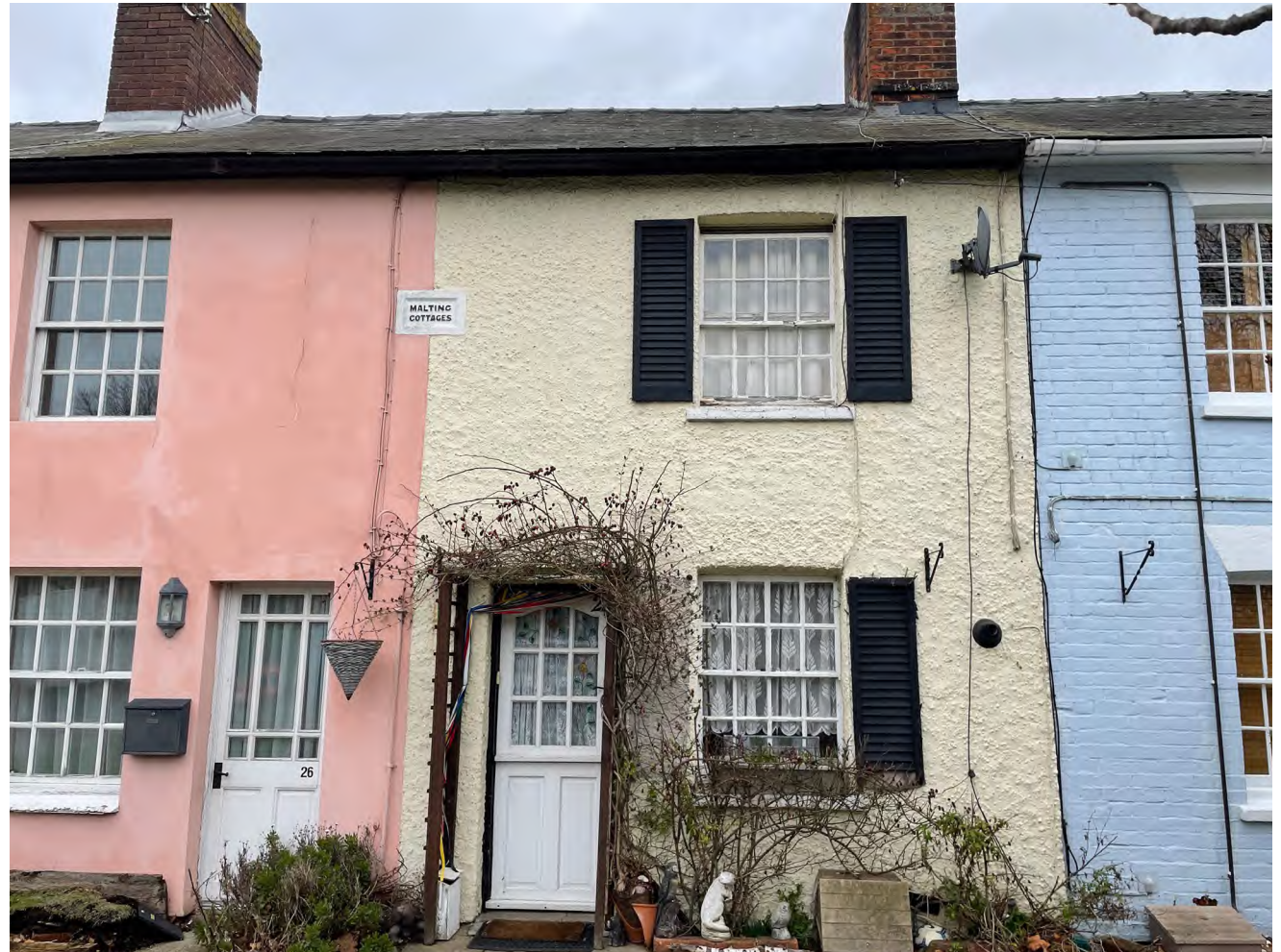
Figure 21 Close up of maltings Cottages
