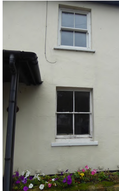
Figure 32 Traditional windows of Number 28 The Street
