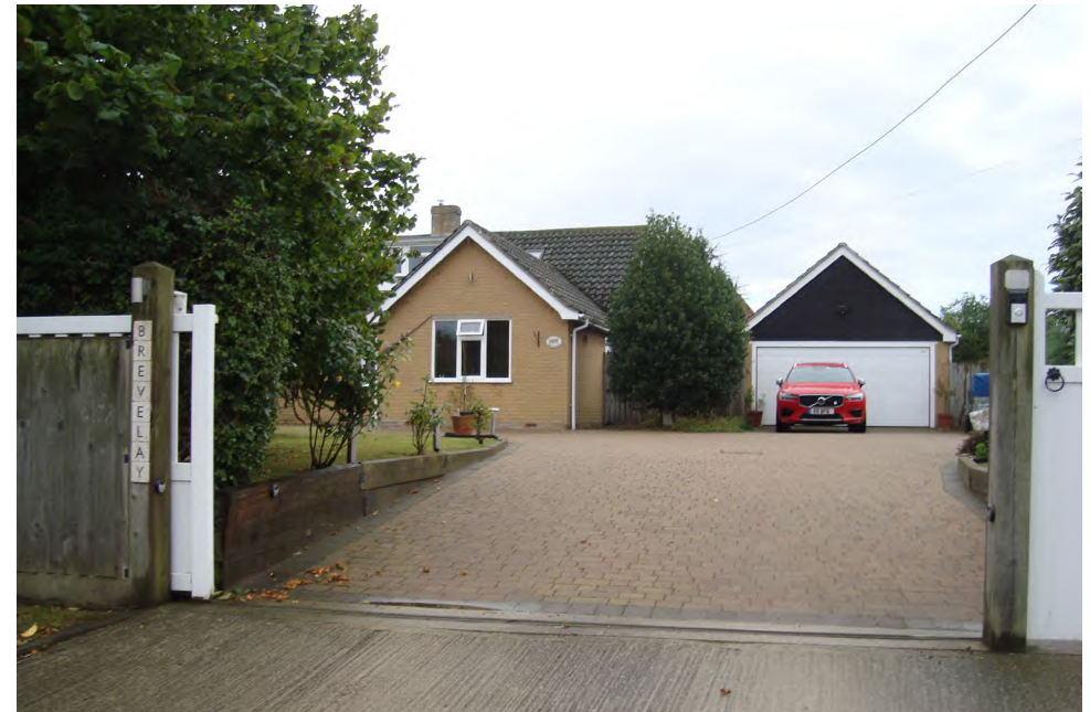
Figure 46 Inappropriate materials including yellow brick and concrete tiles on modern dwellings
