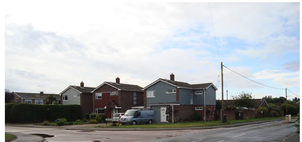
Figure 42 Post-war housing along Hamford Drive forms the setting of the Conservation Area to the west
