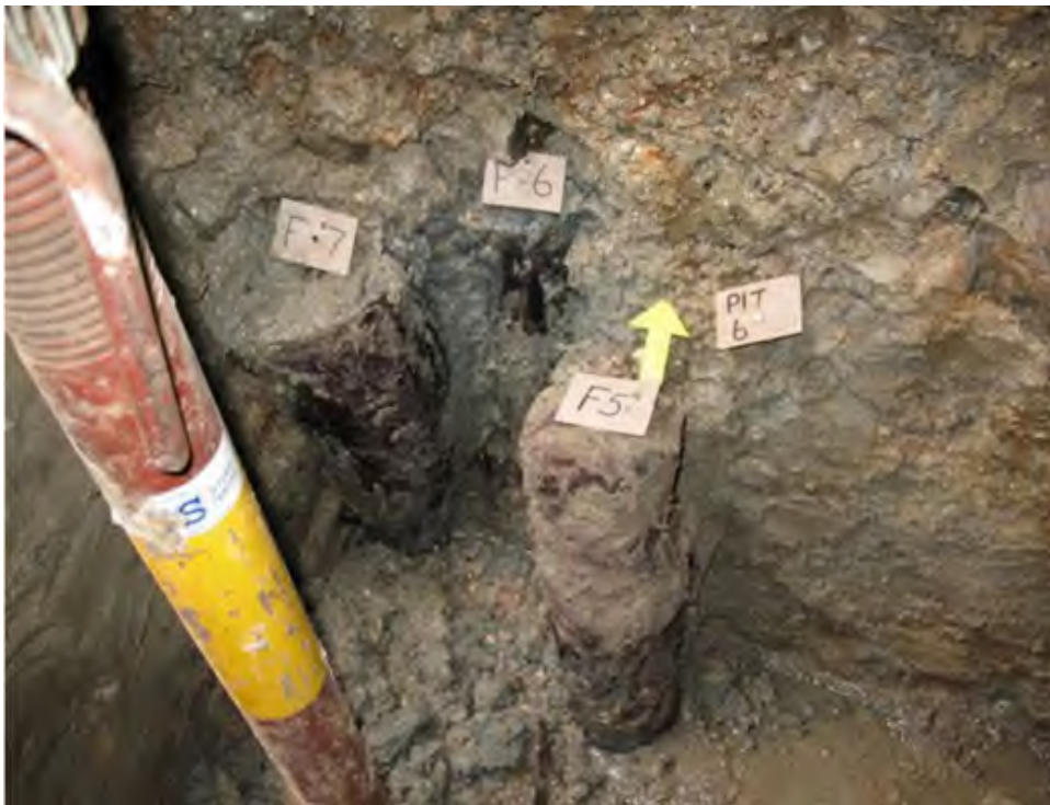
Figure 3 Three wooden piles beneath church tower.
